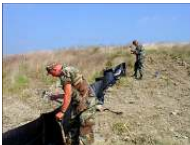
Silt fence maintenance
